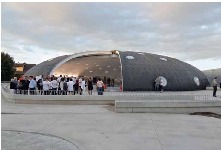
Open roof from outside
