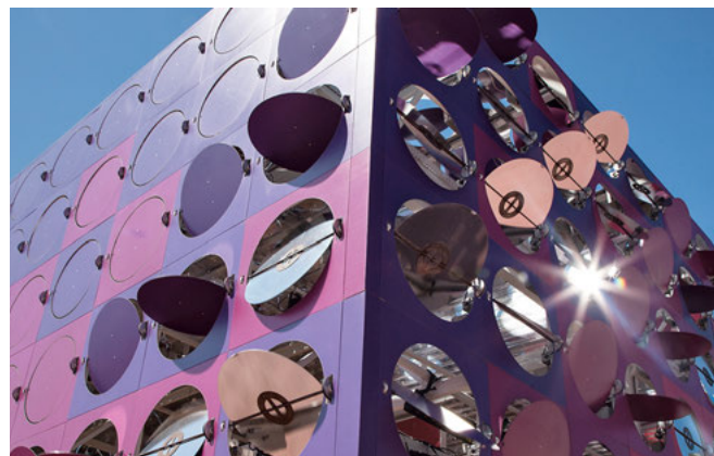
Kinetic facade: metal panels with dancing metal discs
