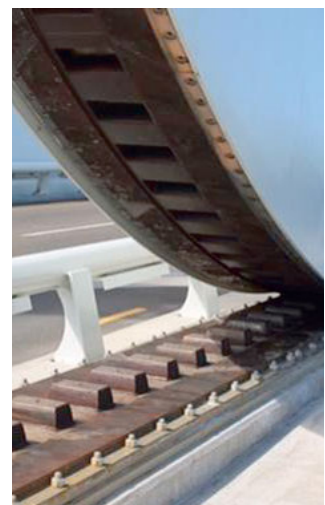
Underside of bridge arm and rack
