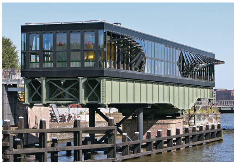
Opening pattern of the folding glazing
