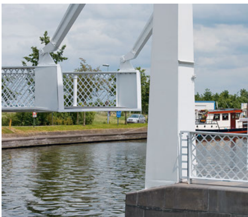
Bridge section (lever arm)
