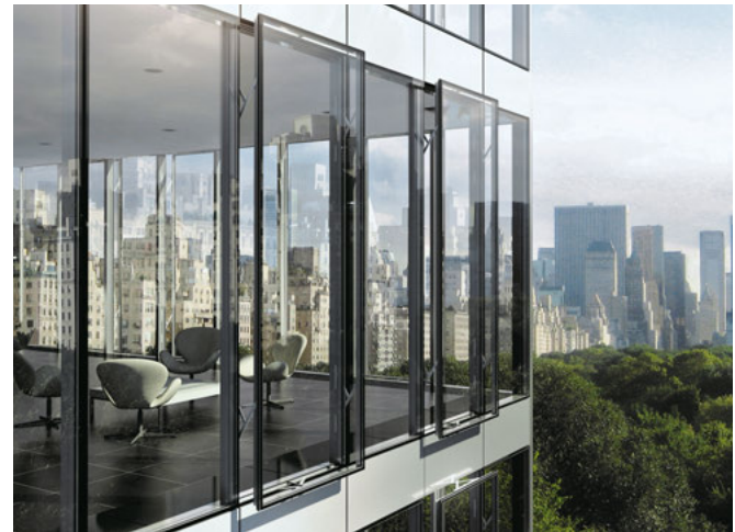
A parallel opening window in a partially open state. Mechatronic fittings allow it to act as a noise insulating vent.
