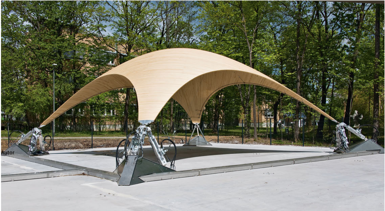
The Stuttgart SmartShell uses computer simulations to precisely model the shell's structural dynamics in advance. The control system uses the results of these simulations to optimise the position of the bearings so that stresses within the material of the shell are kept to a minimum.
