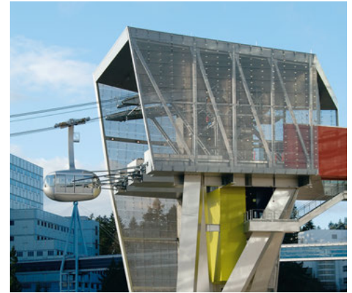
The mountain station is a freestanding tower connected to the existing hospital buildings by a glass bridge.
