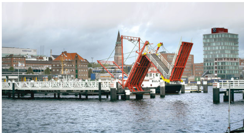
Hörnbrücke in Kiel – a combination of bascule and folding bridge
