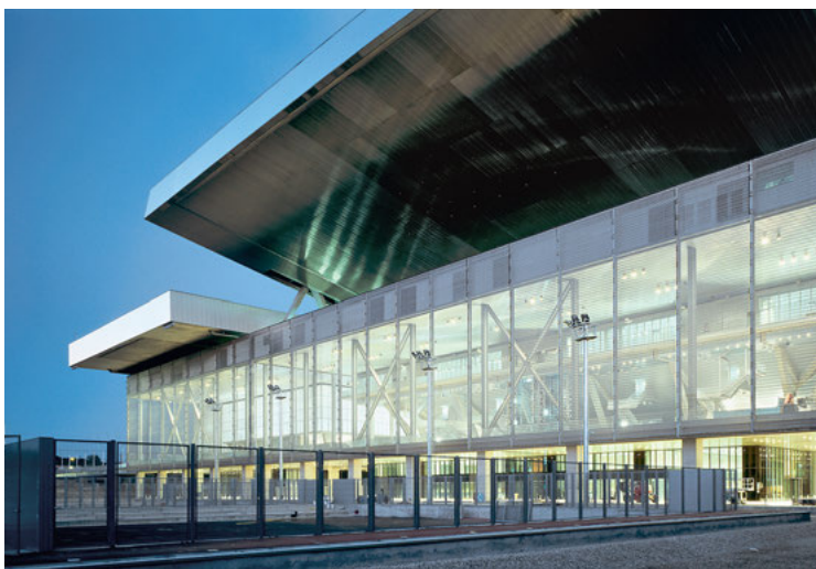
Main roof open
