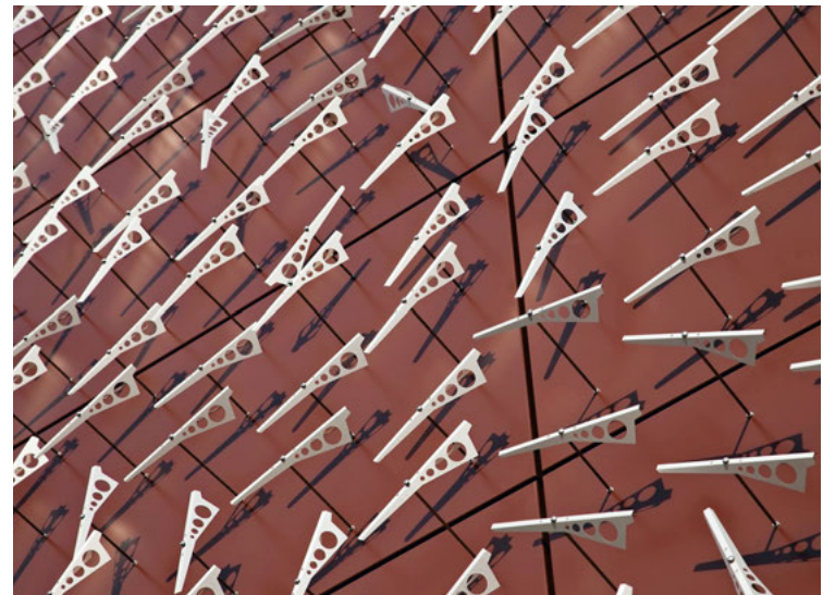
Facade with wind direction indicators
