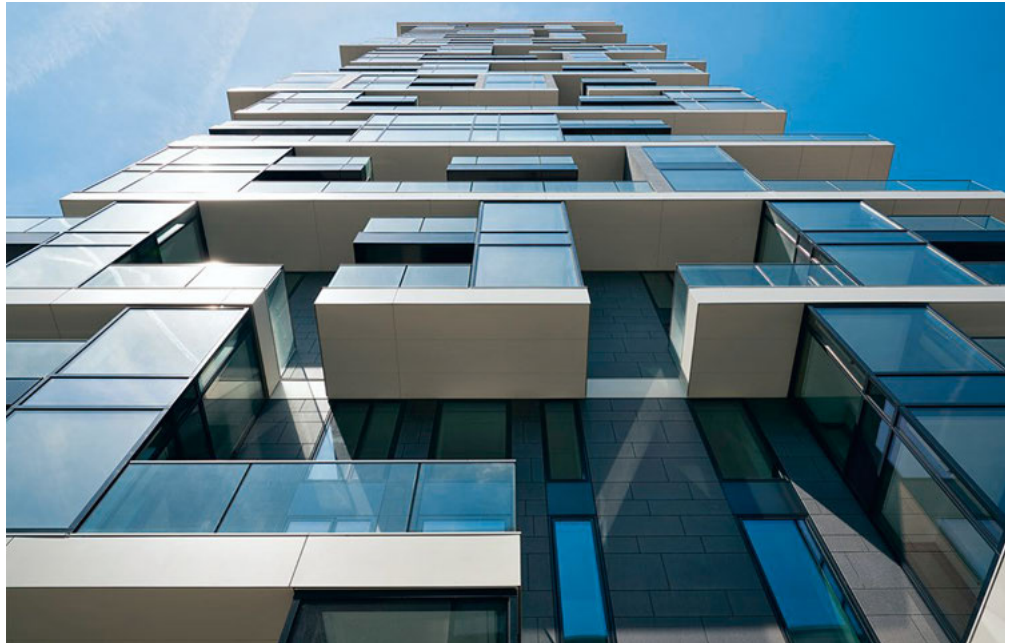
Facade design with surfaces facing in multiple directions developed by WICONA for the new Henninger Turm building, Frankfurt am Main, 2012–2017
