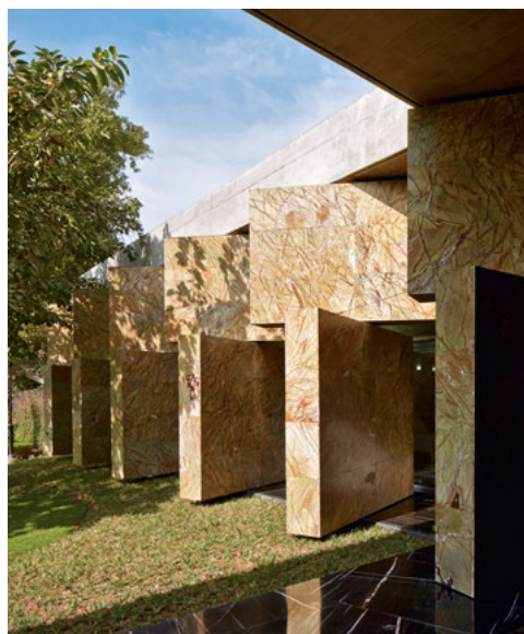
Rotated marble walls
