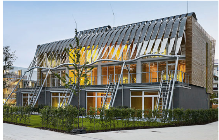
View from the road with 24 m long solar facade
