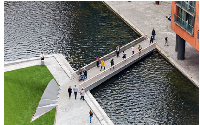
Aerial view of bridge in lowered position
