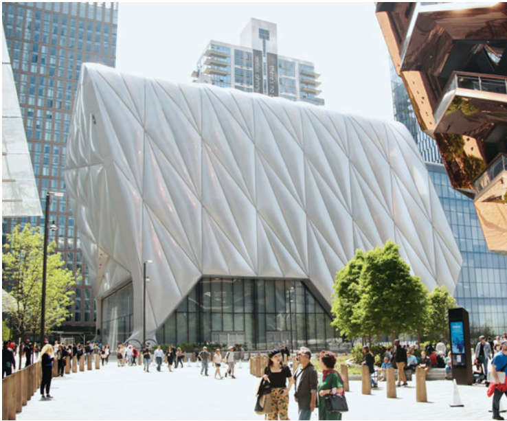
Kinetic building envelope for flexibly programmable space, The Shed, New York City, Diller Scofidio + Renfro, 2018
