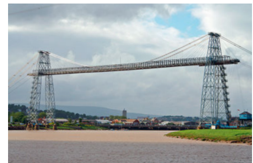
Newport Transporter Bridge
