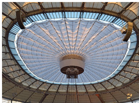
Opening process of the inner roof membrane
