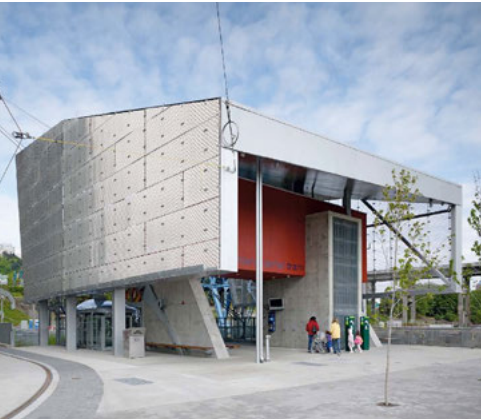
The valley station is an open pavilion seamlessly connected to the public realm.
