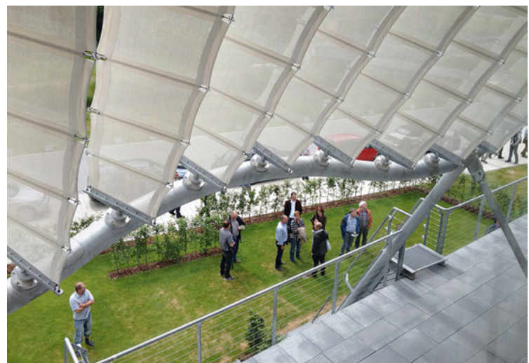
View from above of solar shading strips and terrace
