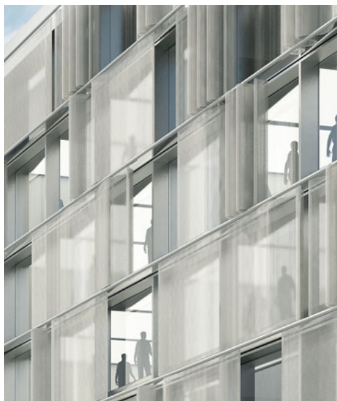
Curved and compressed 3D textiles with transparency control at the macro and meso levels
