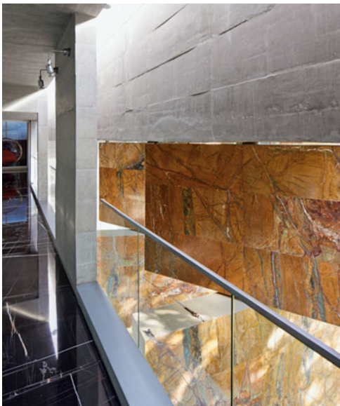
Steel cable connecting the building elements
