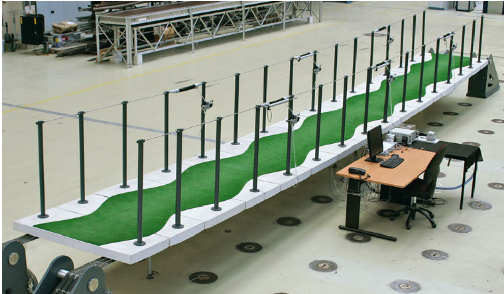
The stress ribbon bridge at TU Berlin, with active vibration control using computer control and six pneumatic muscle actuators in the handrail
