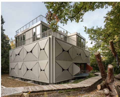
Opening sequence of the facade elements
