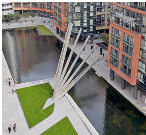
Bridge in raised position
