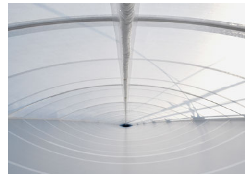
Twin-layer, pneumatically inflated pillows
