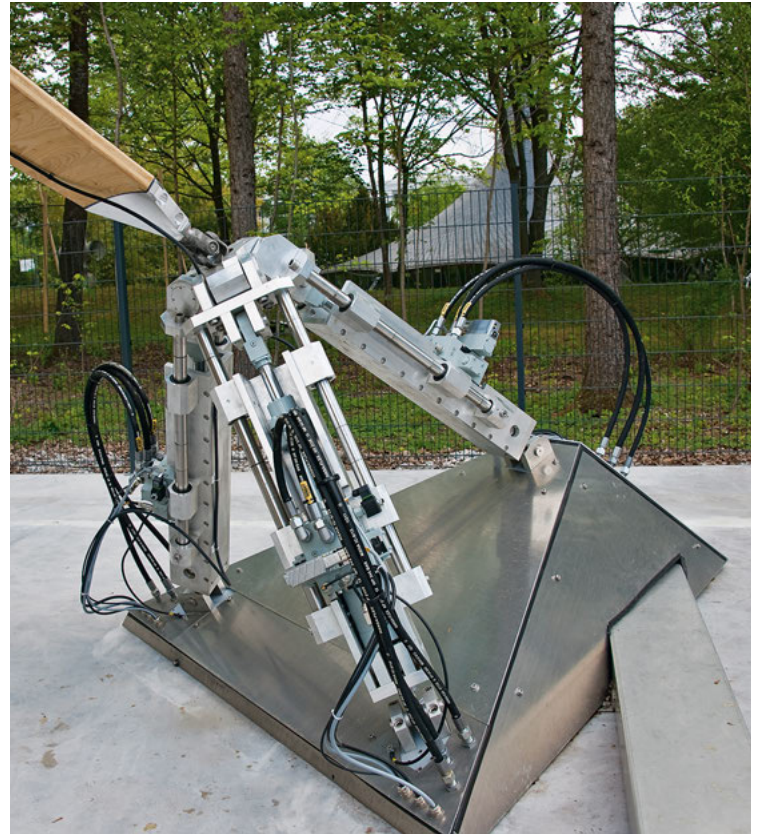
One of the hydraulic bearings of the Stuttgart SmartShell. The system can respond quickly to forces acting on the structure with a degree of accuracy of 2/100 mm.
