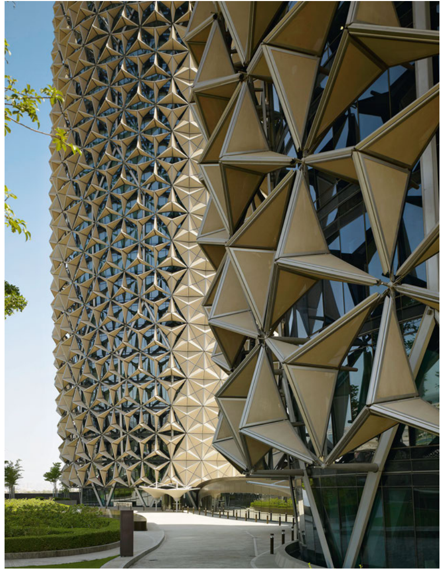
Solar shading system of the Al Bahr Towers, AHR in collaboration with Arup, Abu Dhabi, 2013. PTFE-coated glass fibre mesh mounted on steel supports. Meteorological data on the position of the sun and from sensors are used to control the shading system.
