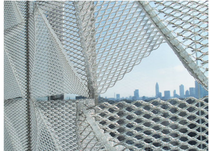
Pleated 3D textiles: hingeless opening mechanism with transparency control at the macro and meso levels
