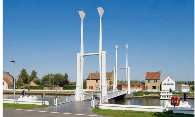
Bridge at rest
