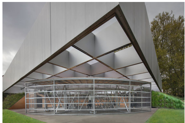
View from outside showing moving element
