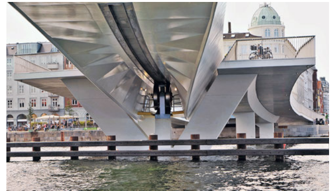
Underside of the drive system
