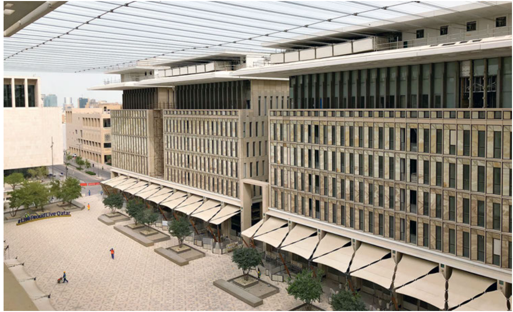
Substructure of the retractable roof
