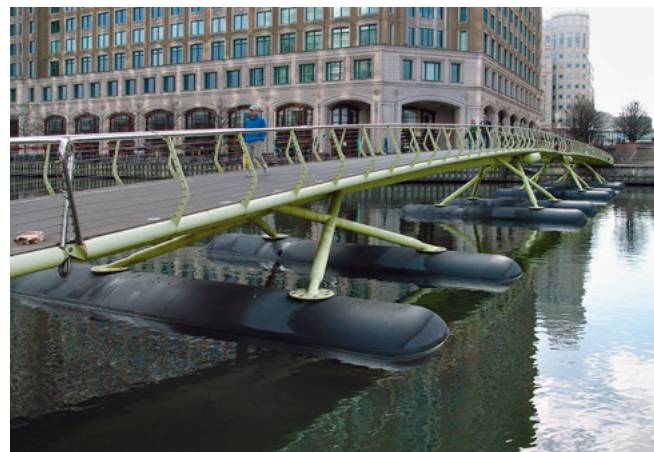
A floating bascule footbridge at West India Quay, London
