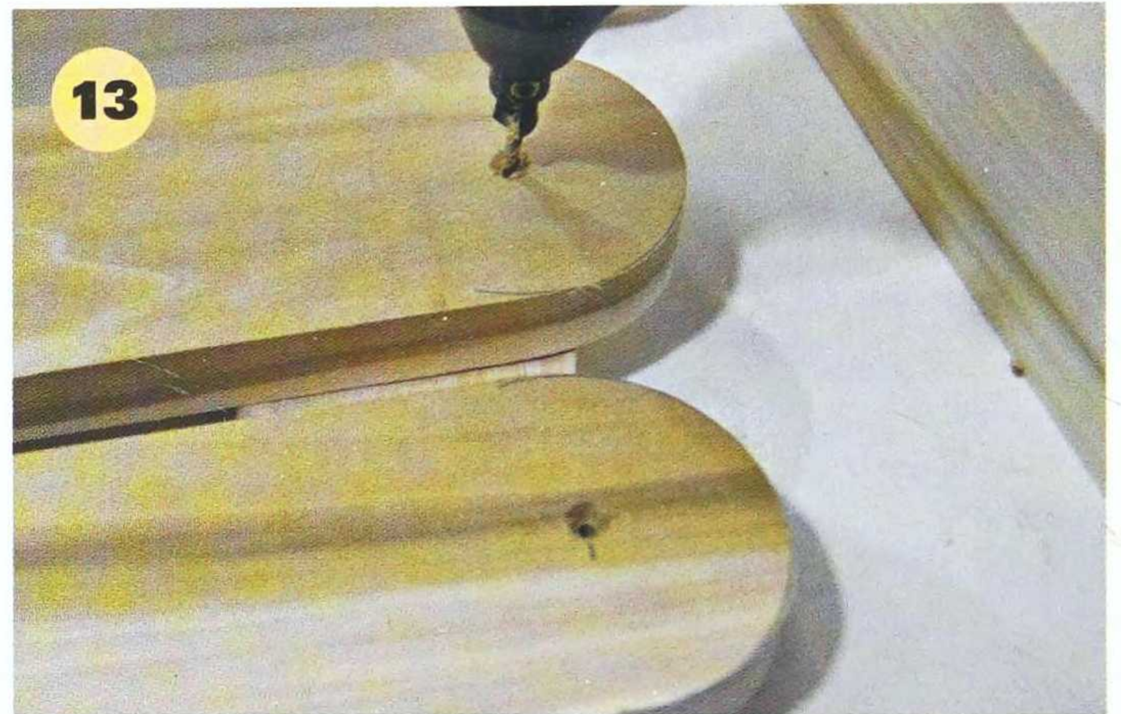
13 Mark and drill the holes for the dowel handle and also cut the radius on the end of the rail.
