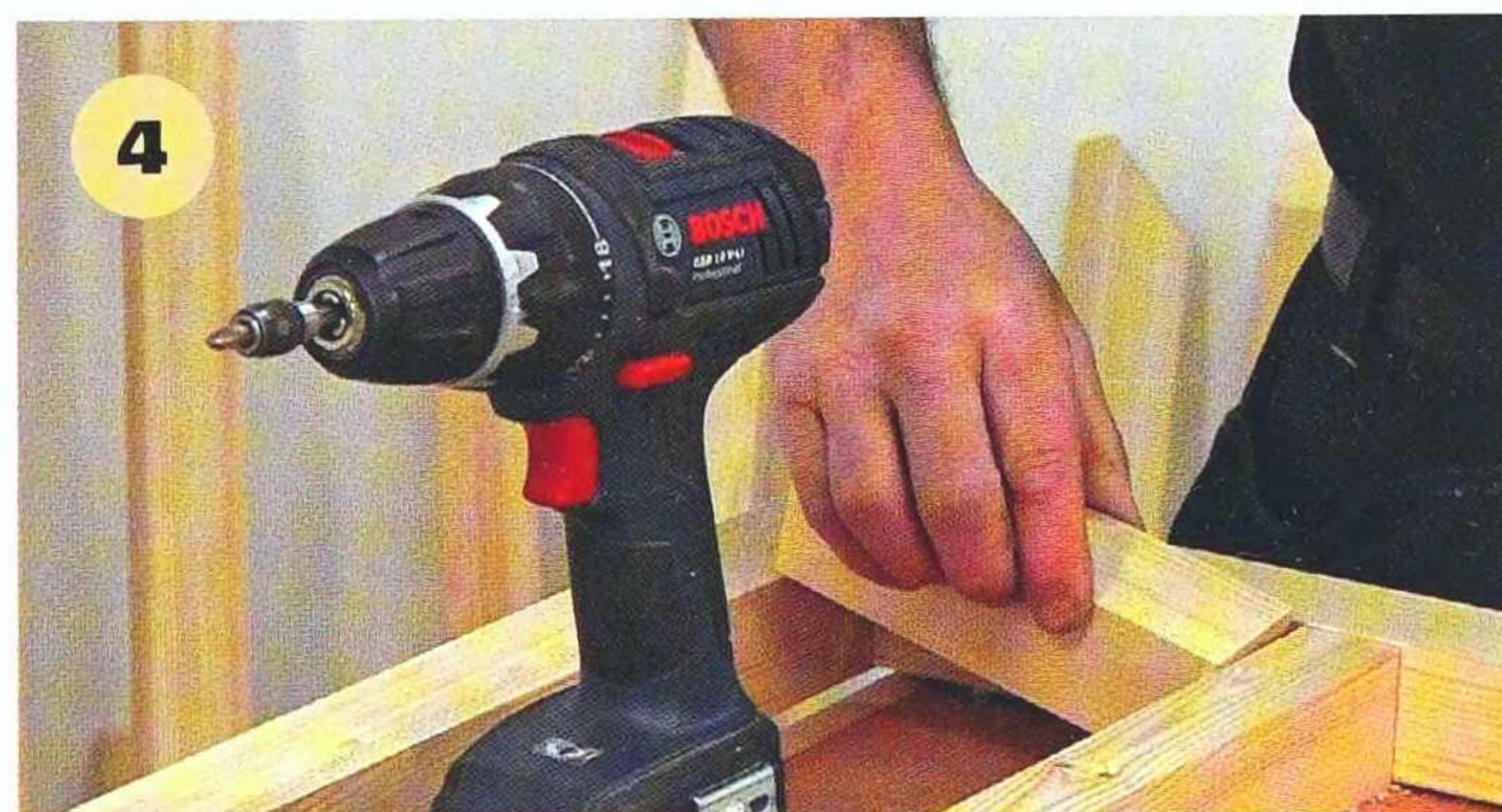
4 Cut a temporary spacer to save measuring for the position of each of the internal uprights.
