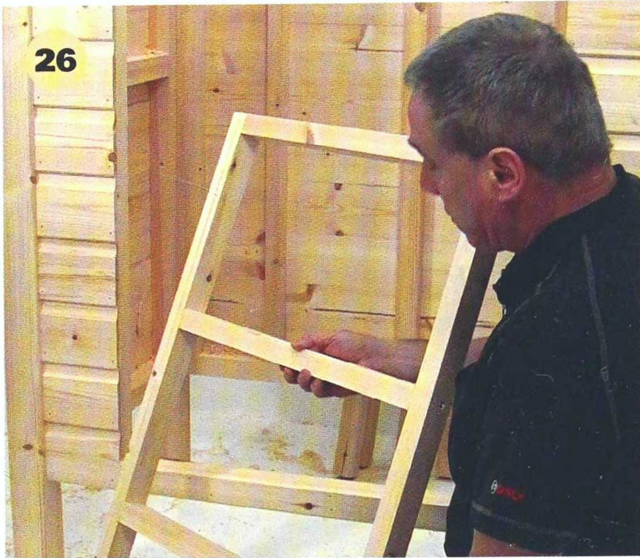
26 Yet another frame is needed for the base; put in a couple of cross bearers to support the plywood floor.
