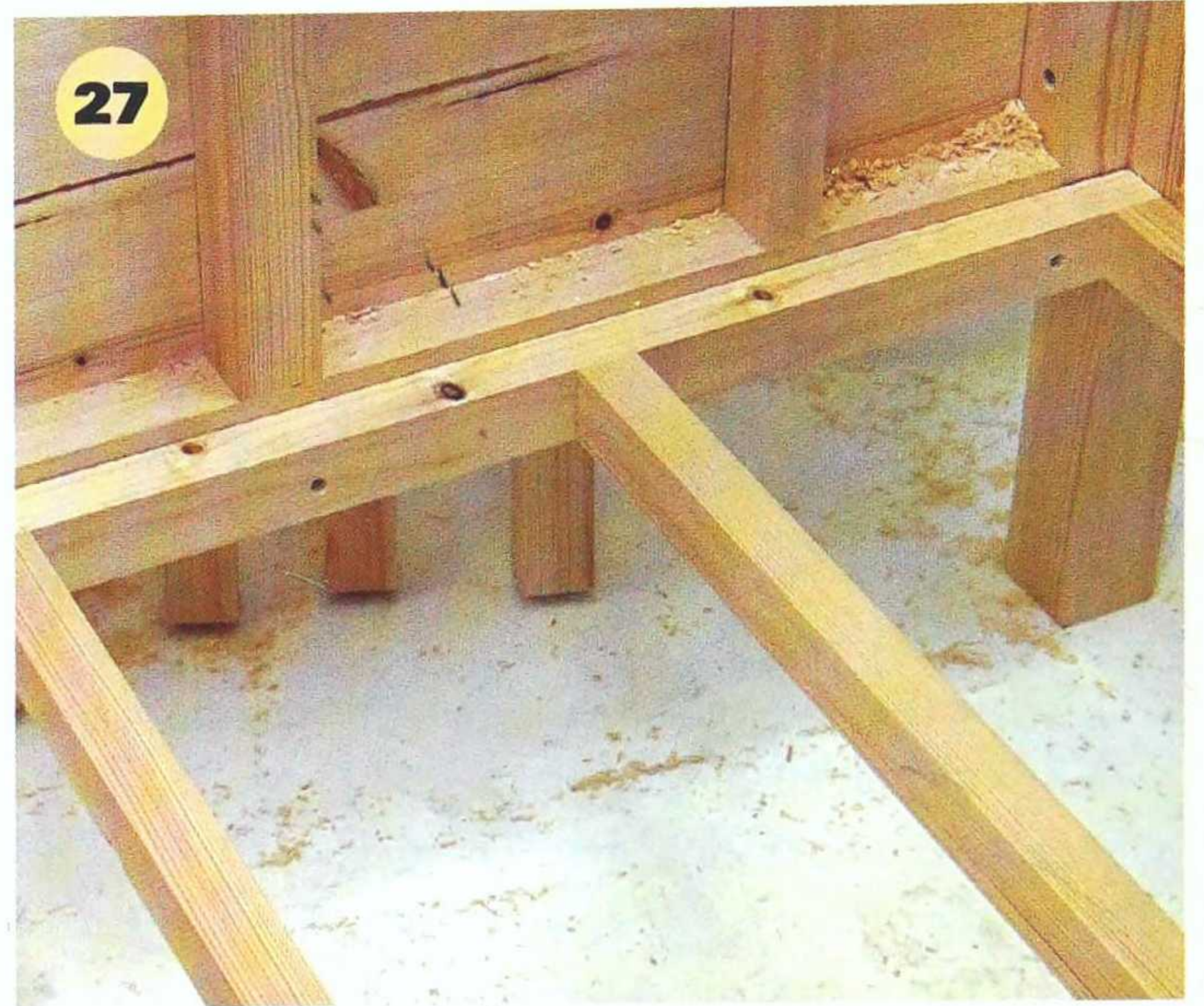
27 This frame is screwed into the base of the shed, but drop it down ½in (12mm) so that the ply base ends up flush with the top of the frame section.
