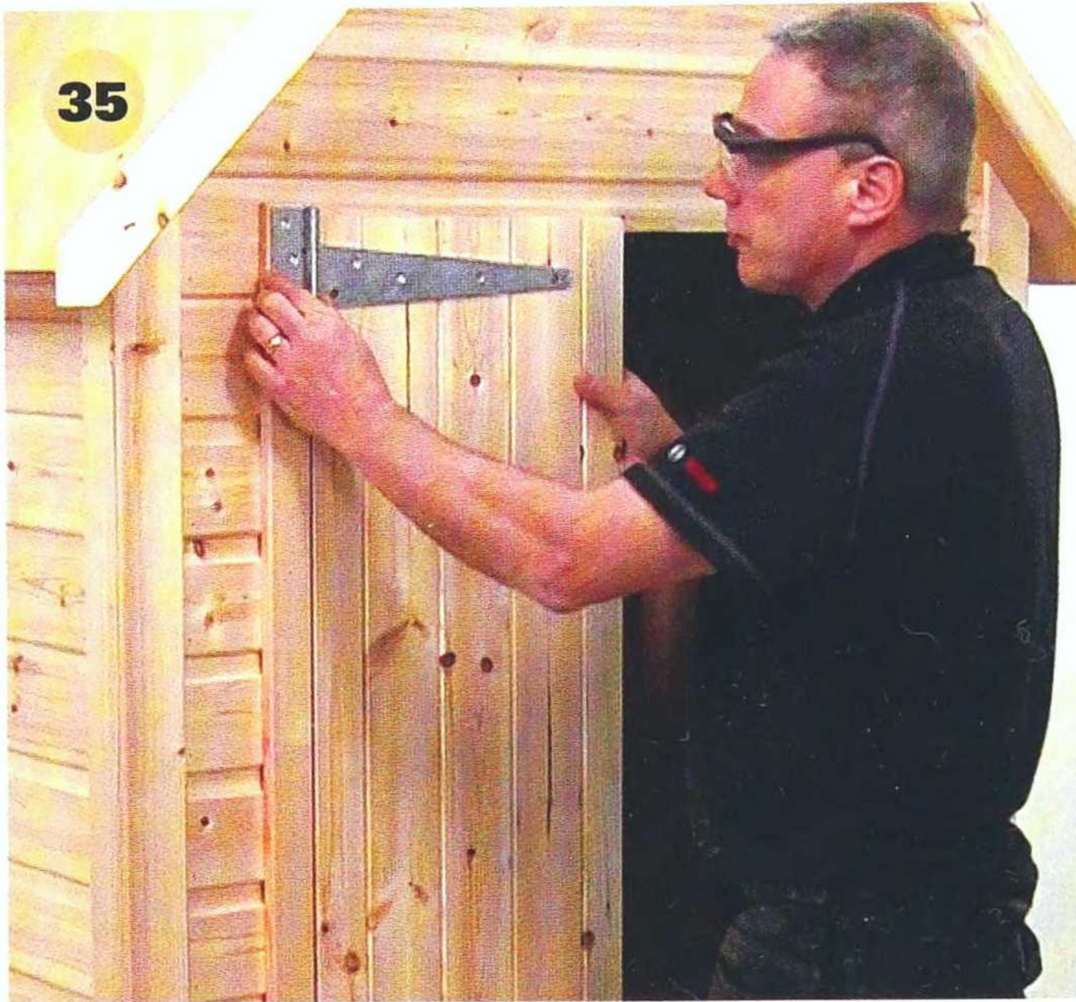
35 Because of the way the doors sit off the front of the shed you will need to fit a packing strip behind them the same thickness as that of the doors.
