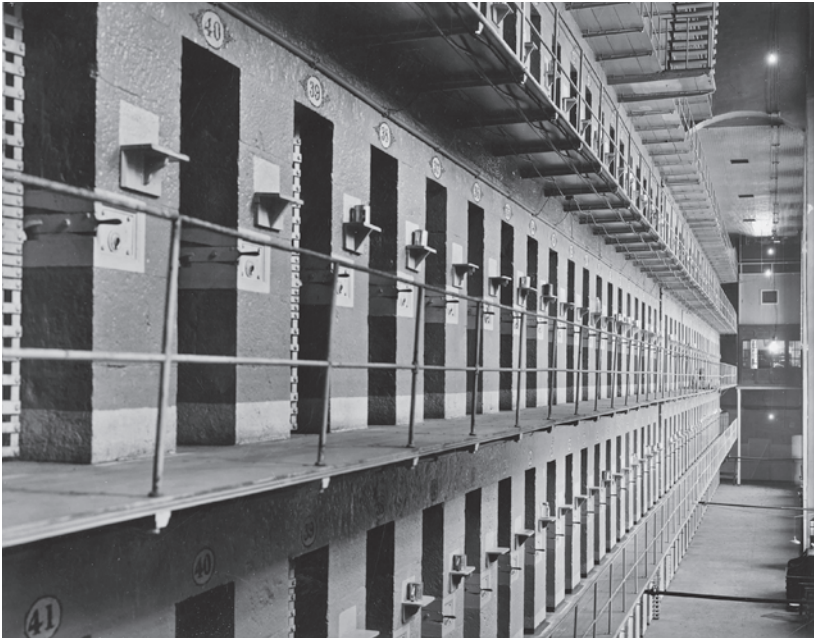
FIGURE 5. Auburn Cell Block in Old South Wing. Photo: Eastern Kentucky University, Correctional Photograph Archives.
