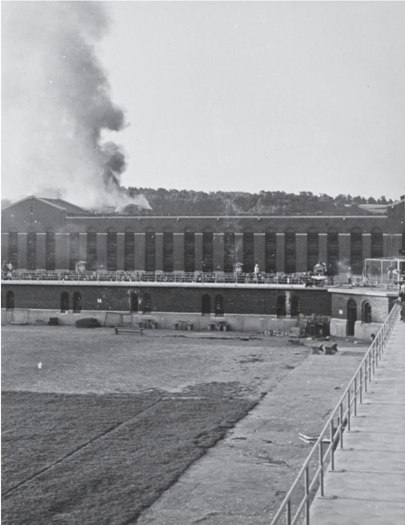
FIGURE 7. Smoke emanating from Attica's chapel. Photo: Attica Brothers Foundation.
