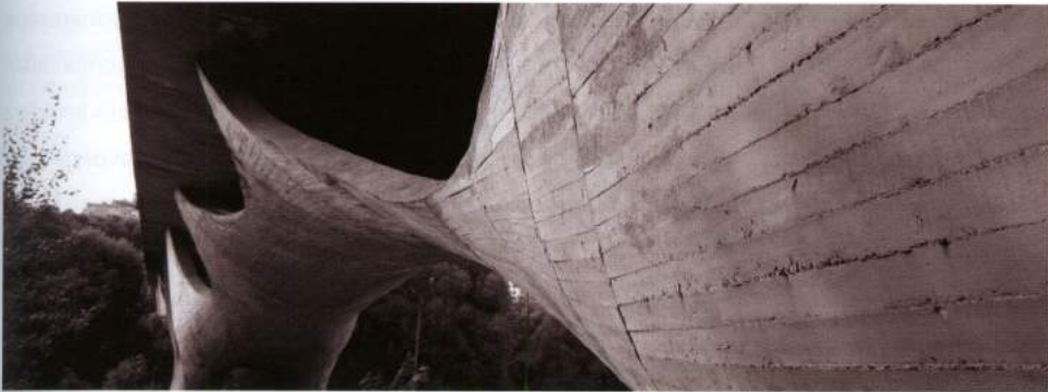
FIGURE 6 Bridge over the Basento River, Potenza (Italy).
