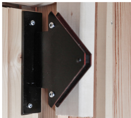
Figure 134. Door closing magnet substitutes more complicated spring-loaded or hydraulic door closer that might not survive for long under sauna conditions.
