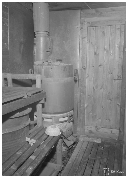
Figure 29. The Finnish Defence Forces led the initiative to create a continuously heated wood-burning heater. The design was based on an existing stove and became housed in a make shift, mobile sauna used for disinfection. Photo: Military Museum, Finland.
