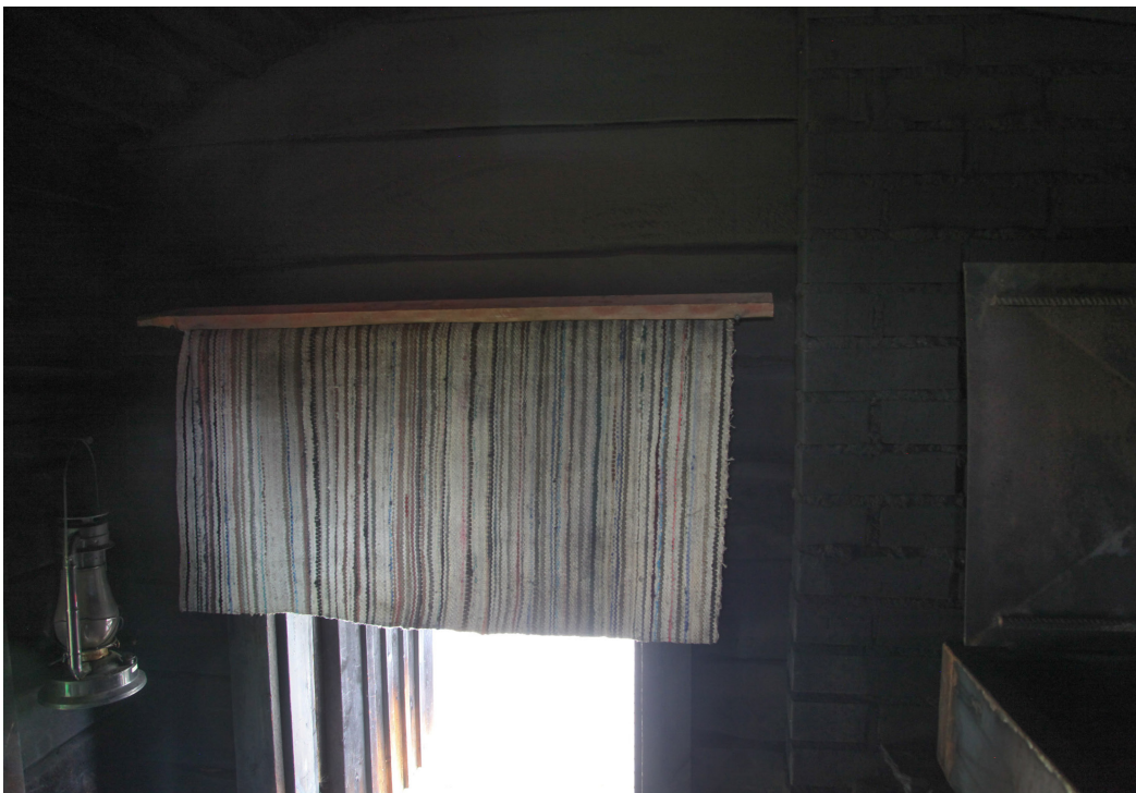
Figure 133. Löyly curtain partially covers the door, minimizing the loss of löyly should the door leak.
