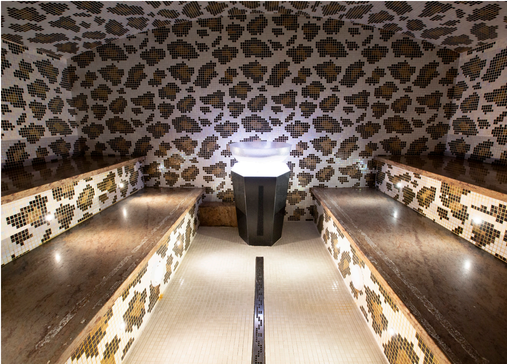
Figure 124. Steam rooms commonly utilize stone or tile seats not common or recommended for sauna.
