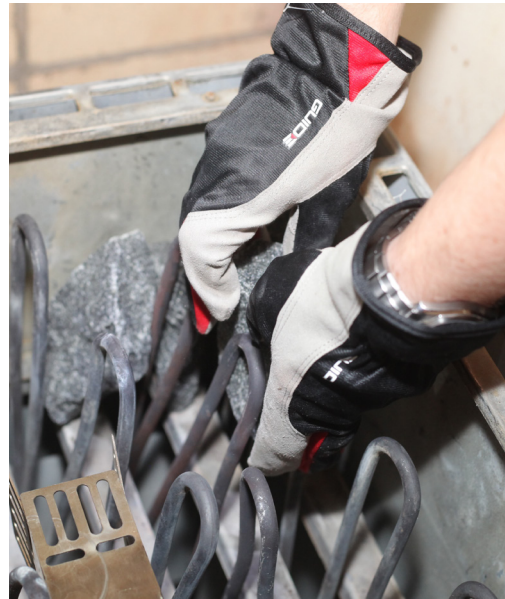
Figure 82. Changing stones to an electric heater.
