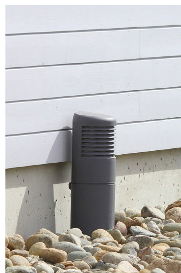
Figure 104. Underground air duct 'Ross' from the outside and the inside of sauna room manufactured by Finnish VILPE. The installation is well hidden from the outside.
