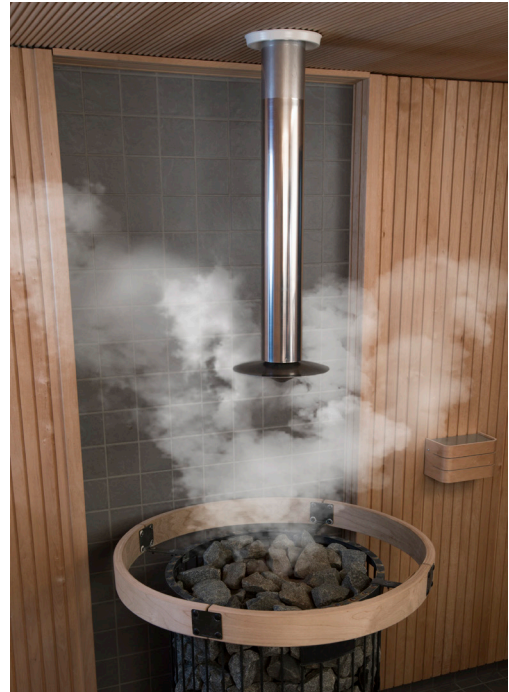
Figure 111. VeskuAir is a Finnish innovation that improves the incoming fresh air flow by leading it closer to the heater and adding a mechanism that prevents löyly from blocking the flow. Photo: © Vesa Leskisenoja.
