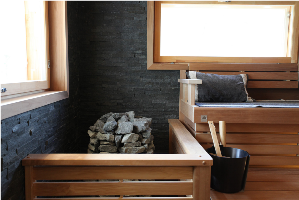
Figure 120. Back support, hand rail, and a heater guard rail made of out alder.
