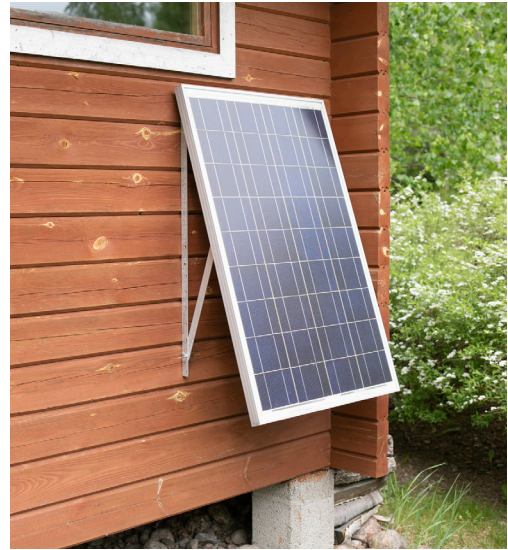
Figure 151. Small solar electricity system is enough to provide energy for lighting in a small off-grid cabin.
