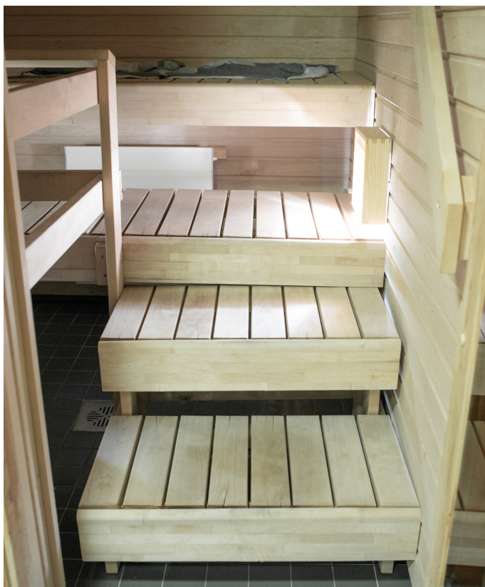
Figure 118. Example bench structure from a typical 4 m 2 electrically heated residential sauna. The elevations starting from the lowest step are approximately +25 cm (10"), +25 cm (10"), +15 cm (6"), and +40 cm (16") raising the top bench altogether 105 cm (42") from the floor. The lowest level of benches in a small sauna is usually a movable stool so it can be easily removed for cleaning.
