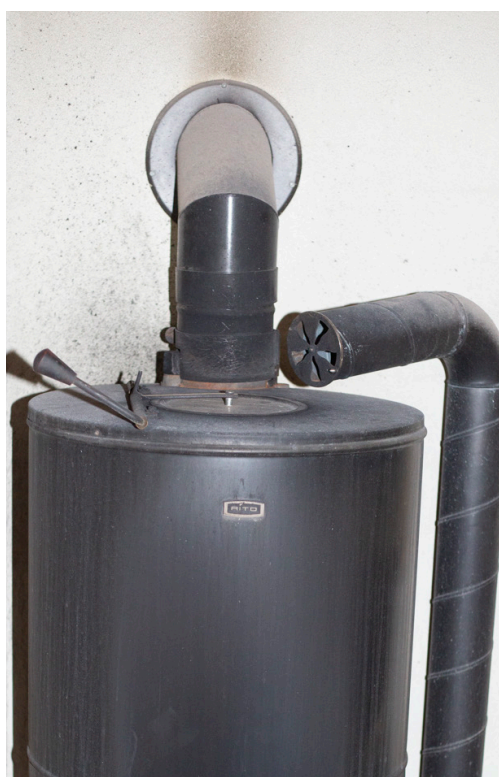
Figure 105. Air duct ending above the top of the heater is recommended.
