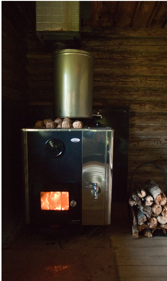
Figure 75. A wood-burning heater with aside and a flue water boiler, potential combined capacity up to 100 liters (26 gallons). Photo © Misa
