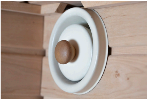
Figure 108. Adjustable vent close to the ceiling is ideal for exhaust as it should be operated everytime sauna is in use.
