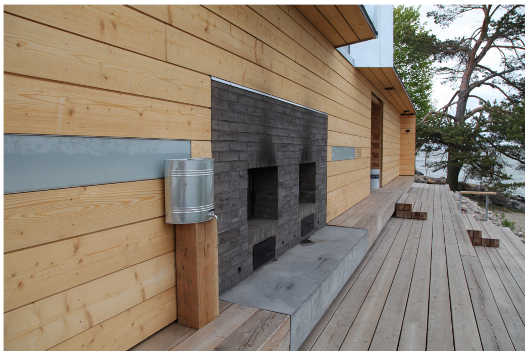
Figure 79. Lonna Island Sauna wood-burning heaters are operated from the outside.
