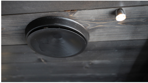
Figure 110. Fresh air vent can be located in the ceiling and is always open.
