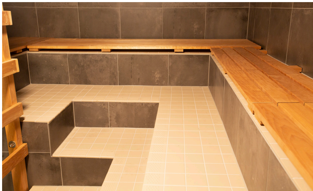
Figure 125. Wooden duckboard covering the tiled bench is a possible solution applied at Uusi Sauna, Helsinki, men's section.
