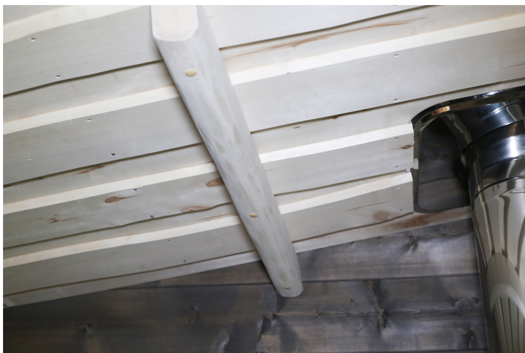
Figure 115. Löyly guide, a piece of wood fixed perpendicularly to the ceiling, in the way of löyly.
