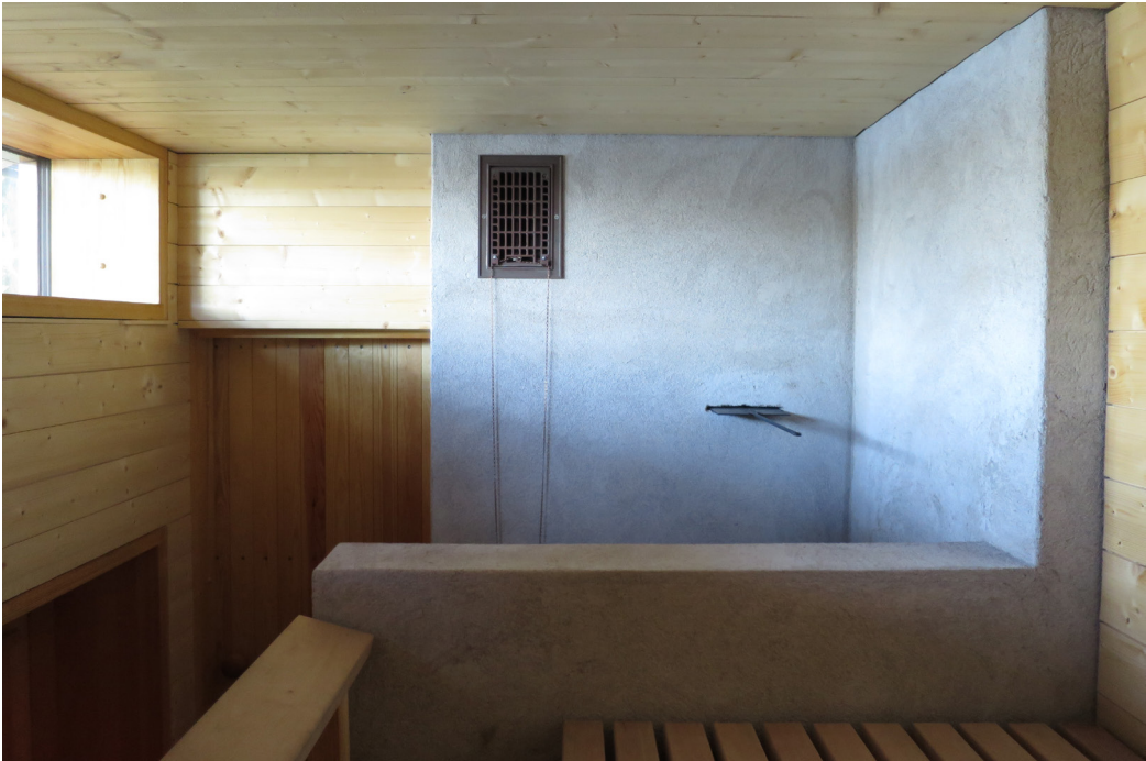
Figure 107. A large vent in connected to a brick flue. (©) Livady Architects
