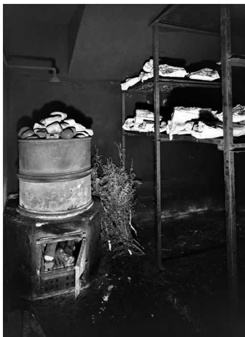
Figure 28. Drum heater ready to go at Elanto sausage factory's smokery in Helsinki. In this case heater operates as a smoke sauna heater without a flue in order. Photo: Helsinki City Museum, 1933. Unknown photographer.
