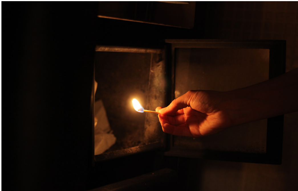
Figure 100. You get the first sense of the ventilation power of the wood-burning heater when you strike a match and see its flame bending towards the fire chamber because of the initial, weak draft.
