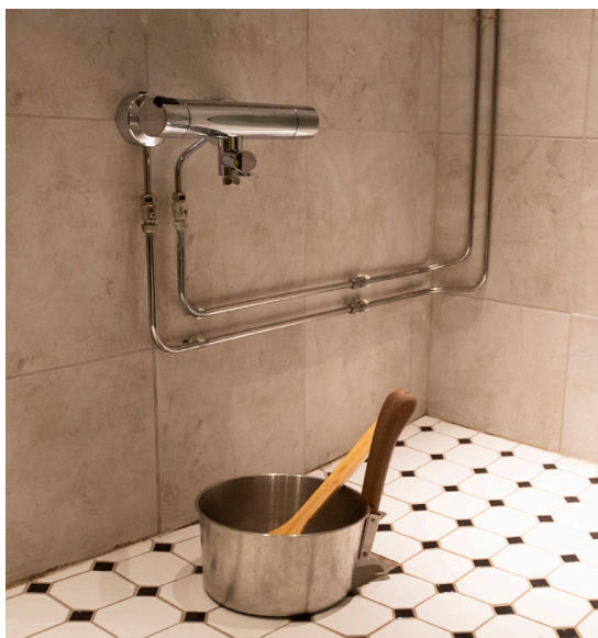
Figure 135. Tiled floor is well-suited for an integrated sauna as long as the tiles have appropriate slip resistance ratings.
