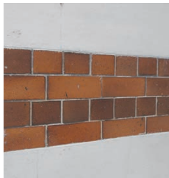
Glazed brick A brick to which a layer of glaze has been applied before firing to give it a different colour and finish.
