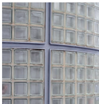
Glass brick Originating in the early twentieth century, glass bricks are usually square. Because they are relatively thick, they provide partial obscuration but still admit natural light into and between internal spaces.
