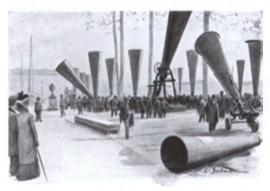
Top left: Nazi engineers developed vortex guns in the hope of incapacitating overflying aircraft by the pressure of sound waves. Hydrogen and oxygen were detonated inside the angled tube of the cannon and projected a plug of compressed air towards enemy aircraft. This example was commissioned by the Reichsluftfahrtamt (Office of Aeronautics) and was used, without effect, to defend a bridge over the Elbe River in 1945. (Author's collection)
