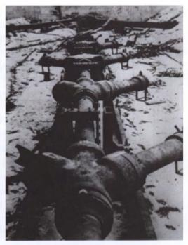
In close view the side-chambers of Hitler's V-3 weapon can be clearly seen. They were designed to fire in sequence to attain maximum muzzle velocity but difficulties in coordinating the explosive charges proved tough to overcome. (Cody Images)
