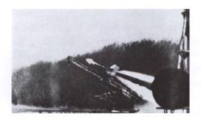
A prototype test flight of the Enzian anti-aircraft rocket developed by Messerschmitt at their Oberammergau research centre. This missile was the first in the world to use infrared guidance systems. (EN Archive)
