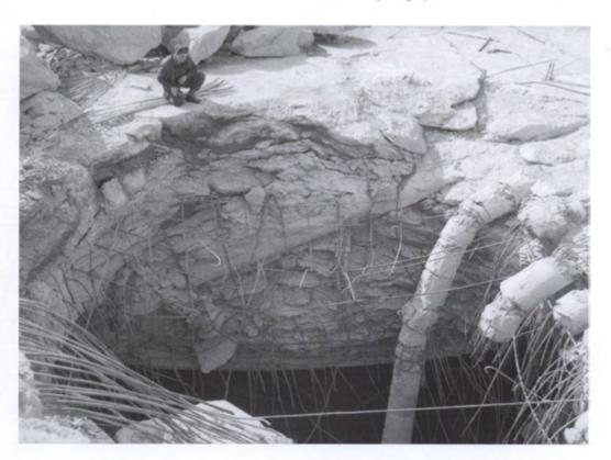
An RAF officer inspects the damage inflicted by a Grand Slam bomb which pierced the reinforced concrete roof of the German submarine pens at Farge, north of Bremen in Germany. This was the result of a daylight raid mounted by 18 Avro Lancasters of No. 617 Squadron on 27 March 1945, in which two direct hits by Grand Slams led to the collapse of the partially completed roof. (IWM CL 2607)
