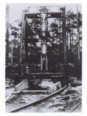
An A-3 rocket mounted at Kummersdorf on stand no. 3. This was the largest at Kummersdorf and could be moved along the rails that can be seen in the photograph. (Science Photo Library)
