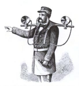
A Victorian woodcut shows the topophone, invented and patented by Professor A. M. Mayer in 1879 and featured in *Scientific American* in 1880. The instrument was designed to amplify noises and help the listener determine their exact direction. (© Bettmann/Corbis)
