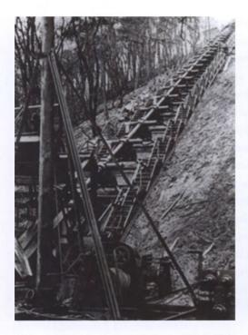
The V-3 was an extended gun with side-chambers that fired in sequence to project a shell over 100 miles (160km). It was fired against London and Luxembourg in 1944 and 1945. (Author's collection)
