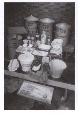
This photo from 1941 shows the equipment that was assembled to decontaminate gas casualties at a cleansing centre in London. Efforts on the Home Front helped ensure that England's civilian population would be well-placed to cope with poison gas attacks. (IWM D 3925)
