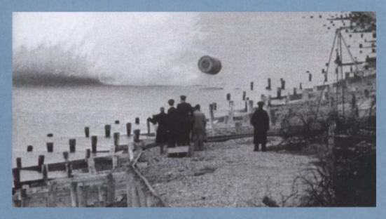
Prior to Operation Chastise, No. 617 Squadron practised dropping the Upkeep weapon at the Reculver bombing range on the Kent coast. Observers keep watch as the bomb bounces toward the shoreline. Barnes Wallis, on the extreme left of the group, seems to be urging the weapon on to success. (IWM FLM 2343)
