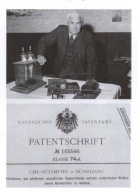
Christian Hülsmeyer demonstrated that remote detection of objects was possible. He is here seen with his patent for the Telemobiloscope dating from 1904. (akg-images/ullstein bild)
