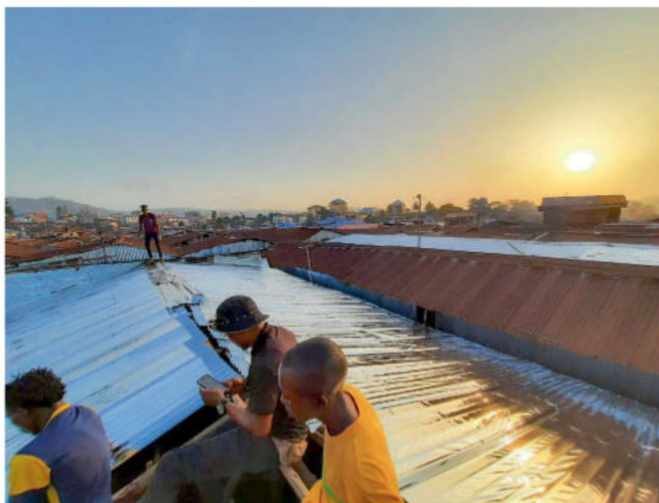
Mirrored film on two roofs in Sierra Leone (above) made it cooler inside. The roofs (right-hand pair of rectangles in top-right image) show up darker, so cooler, on a heat map
