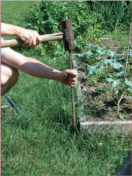
Driving the rebar into the ground.
