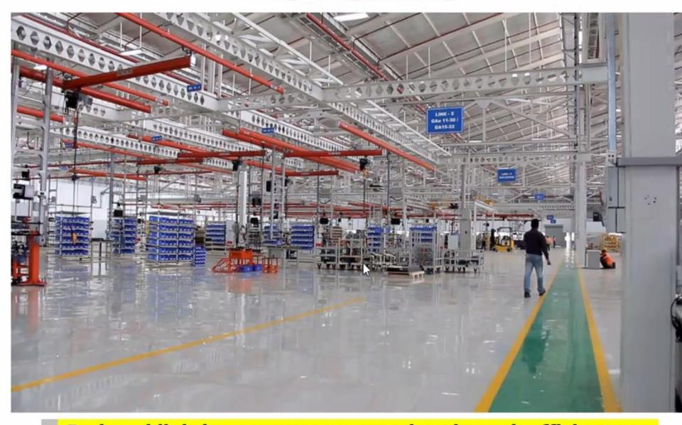
Reduced lighting energy consumption through efficient use of skylight and light pipes
