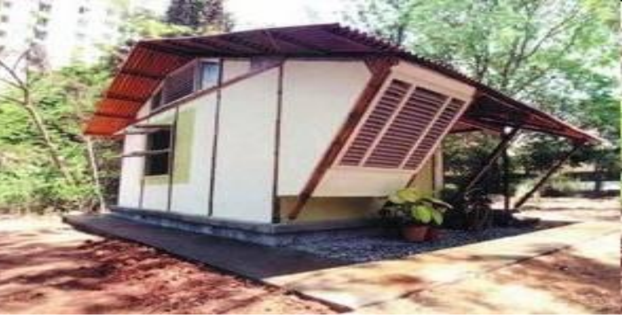
BAMBOO HOUSES WITH BAMBOO MAT
