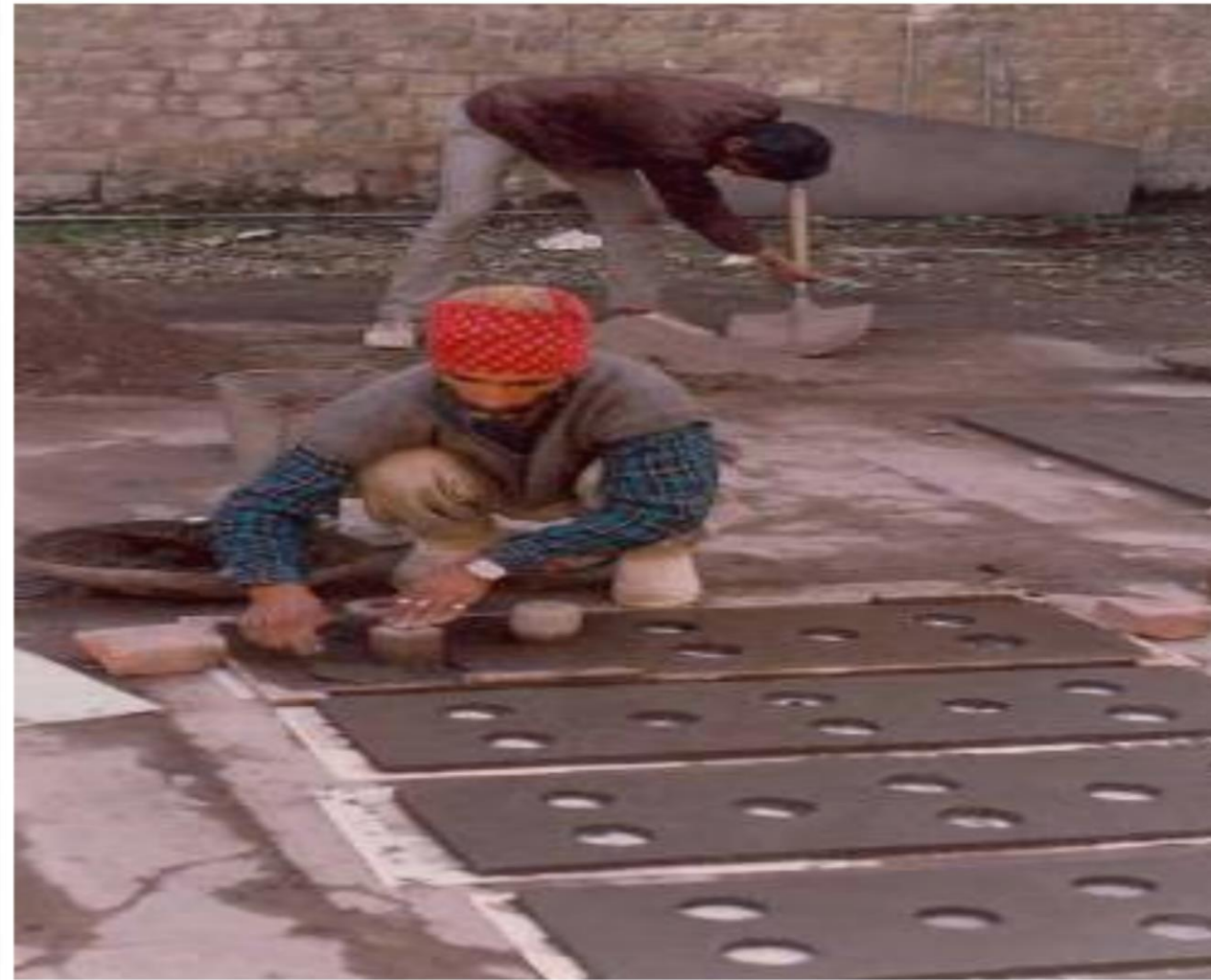
Construction of Ferro-cement Columns and Slabs
