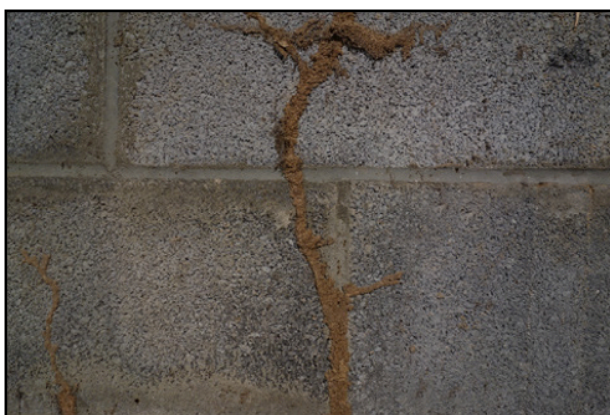
FIGURE 18-3: Termite mud tunnels on a house foundation.
