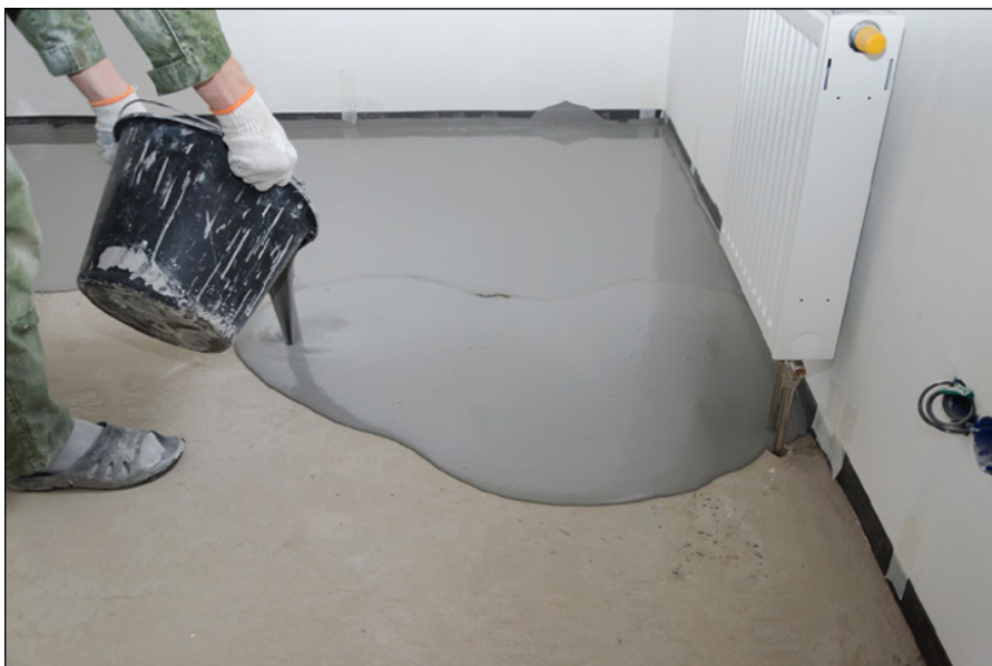
FIGURE 4-12: Floor-leveling compound being poured across a floor.
