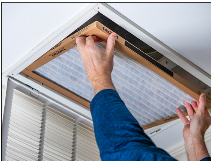
FIGURE 10-2: Replacing a dirty HVAC filter at a ceiling return register.
