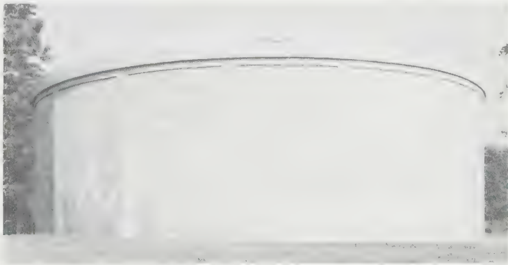
FIG. 35. Prestressed-concrete water-storage tank. ( Natgun. )
