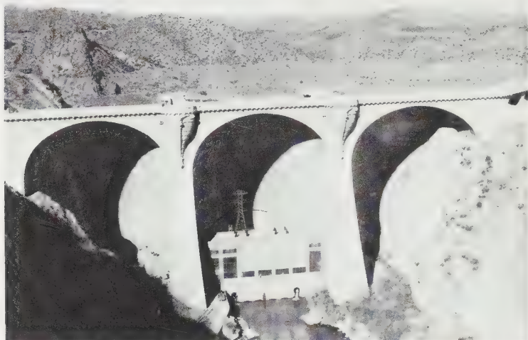
FIG. 5. Coolidge Dam, general view—multiple-dome type.
