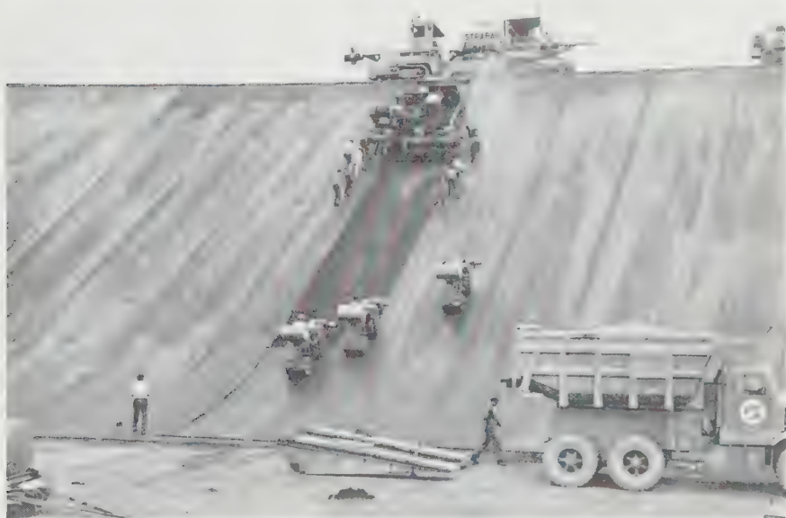
FIG. 4. Placing upper-reservoir bituminous lining at Vianden.
