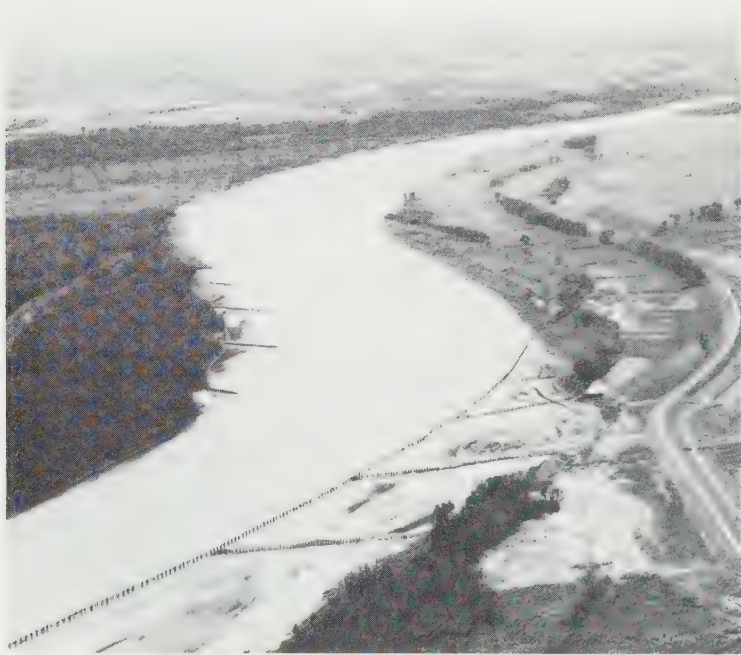
FIG. 7. Realigned channel before accretion.
