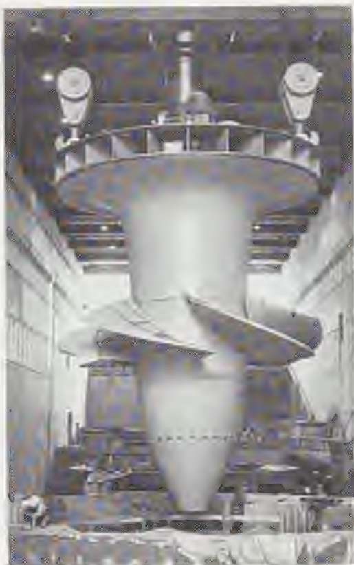
FIG. 13. A runner, shaft, and head cover assembly being lowered into the turbine pit of one of the 114,000-hp Kaplan turbines in the Priest Rapids powerhouse. Weight of assembly 750,000 lb. ( English Electric Company Ltd. )
