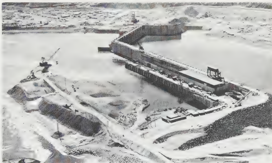
FIG. 14. Wanapum Dam project (Washington)—river diversion.
