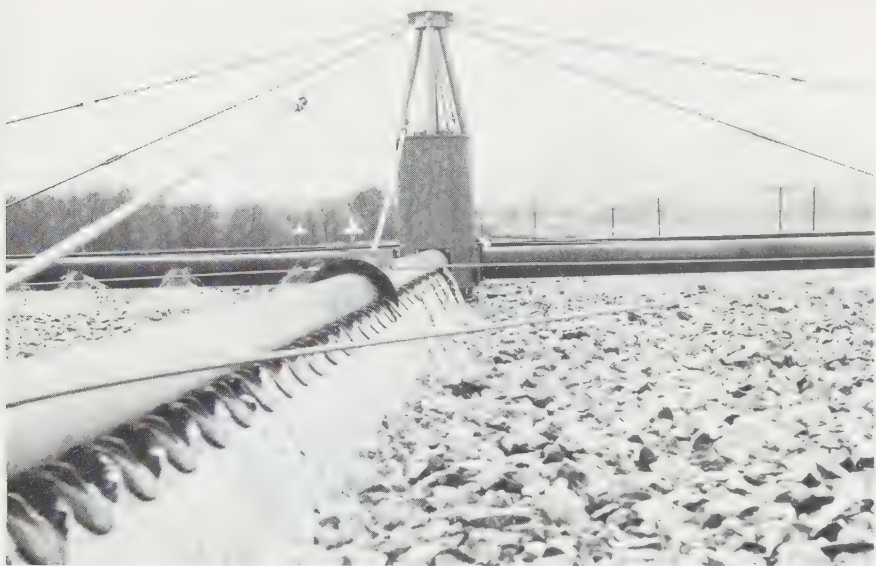
FIG. 15. Rotary distributor for trickling filter. (Yeomans.)
