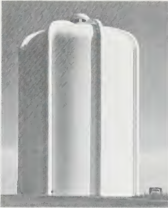
FIG. 34. A 3-million-gal standpipe with ornamental cupola and pilasters in Madison, Wis., 73 ft in diameter by 90 ft high. ( Chicago Bridge and Iron Co. )
