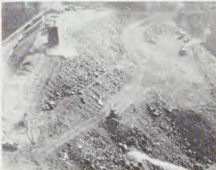
FIG. 6. View of New Exchequer Dam—rock-fill construction.
