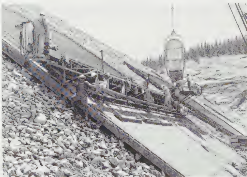
FIG. 8. View of Cabin Creek Dam —placing of concrete face (engineer—Stone & Webster Engineering Corp.; contractor—J. A. Jones and P. Harrison).
