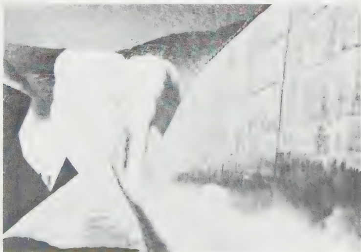
FIG. 22. Derbendi Khan Dam—spillway and bucket in action.
