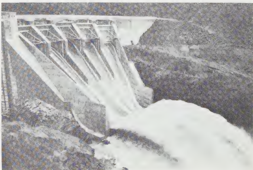
FIG. 40. Mayfield—initial operation under partial gate openings.
