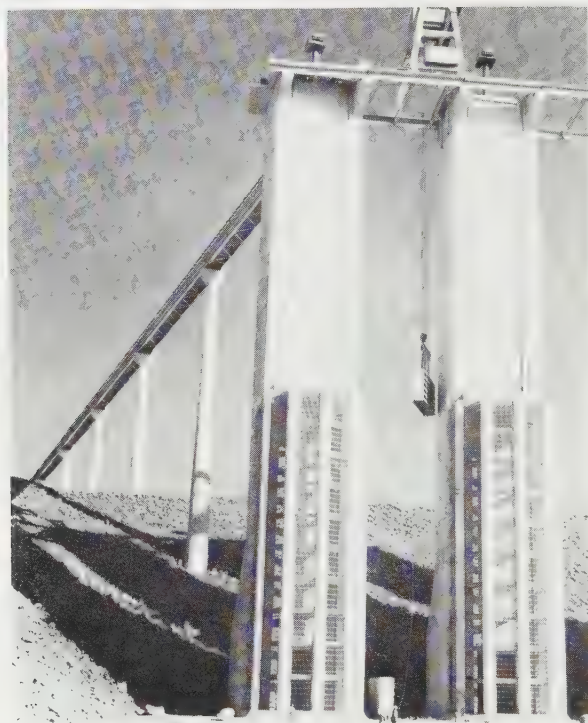
FIG. 4. Tower intakes at San Luis Dam in California. Note lifting frame and bulkhead gate section being hoisted by gantry crane for storage on the tower service deck.
