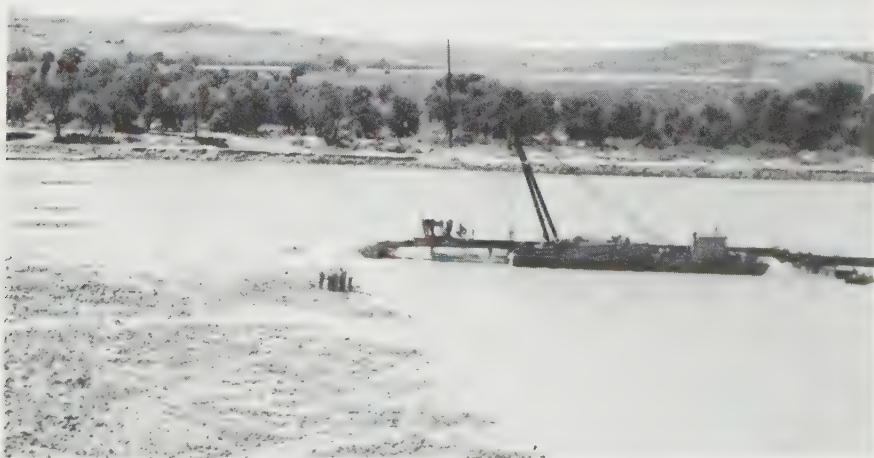
FIG. 12. Closure of river at Fort Randall Dam (South Dakota).
