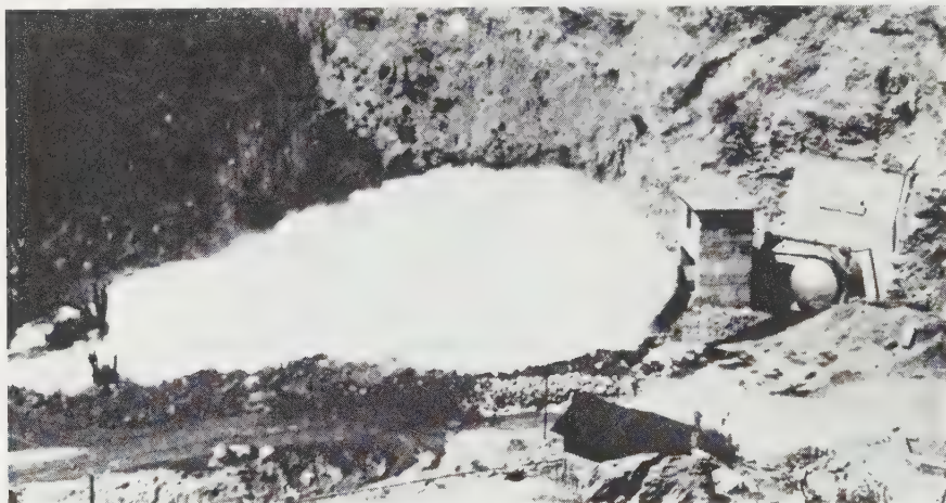
Fig. 32. Free discharge from 54-in. Howell-Bunger valve under 138-ft head. ( Allis-Chalmers Manufacturing Company. )
