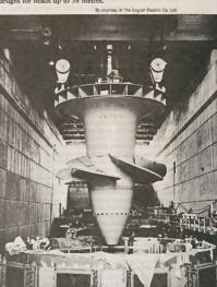
Figure 5: A 131,000-horsepower Kaplan water-turbine runner
