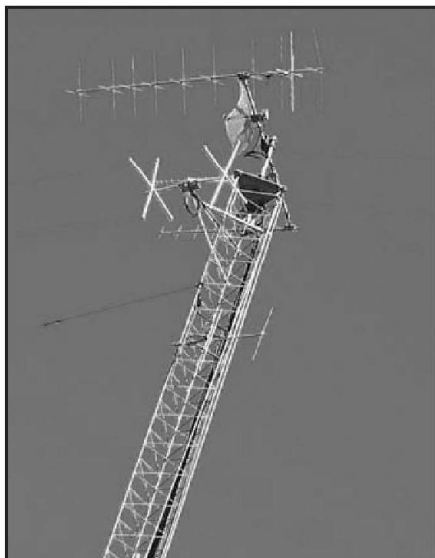
Figure 2—Looking up the tower at the center spreaders of the Cage antenna at W1AW.
