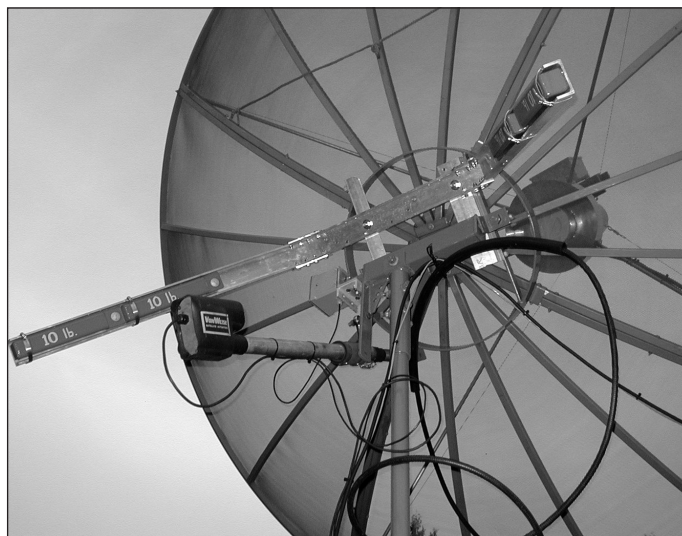
Figure 74 — Mounting arrangement, counterweights and az/el control system for the VA7MM 3 meter dish.
