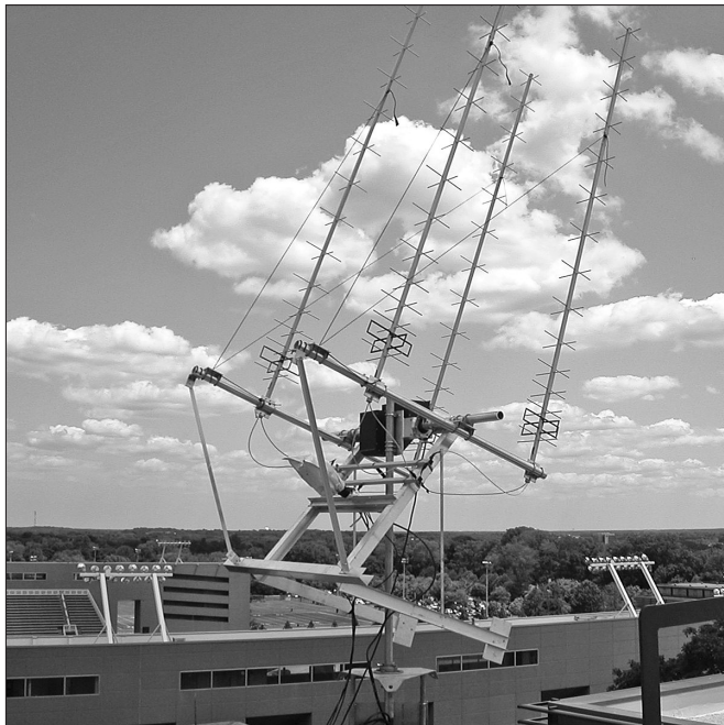
Figure 72 — Dual-polarization EME array at W2PU. At the left, shows the four 15-element, rear-mounted Yagis. Boom length is 3.5 m, and stacking distance is 1.2 m in each direction. The right photo is a close-up showing some details around the driven loops.
