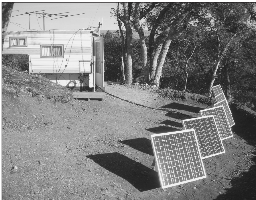
Figure 24.53 — Solar panels can be used to charge a bank of batteries to supply power. Effective off-grid power requires an accurate and conservative estimate of power needs and available energy sources. [Rick Hilding, K6VVA, photo]
