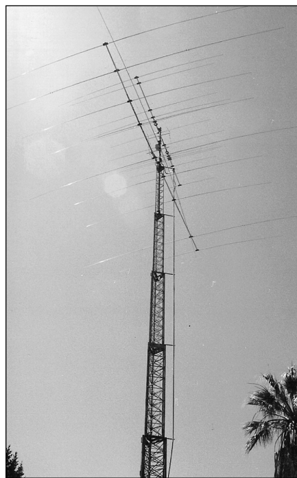
Figure 22.11 — The bottom of a crank-up tower is shown at left. The motor drive mechanism is on the left and a fishing net on the right catches and coils the feed lines and control cables as the tower is lowered. On the right, a fully loaded crank-up extended to its maximum height of 90 feet. [Steve Morris, K7LXC, photos]
