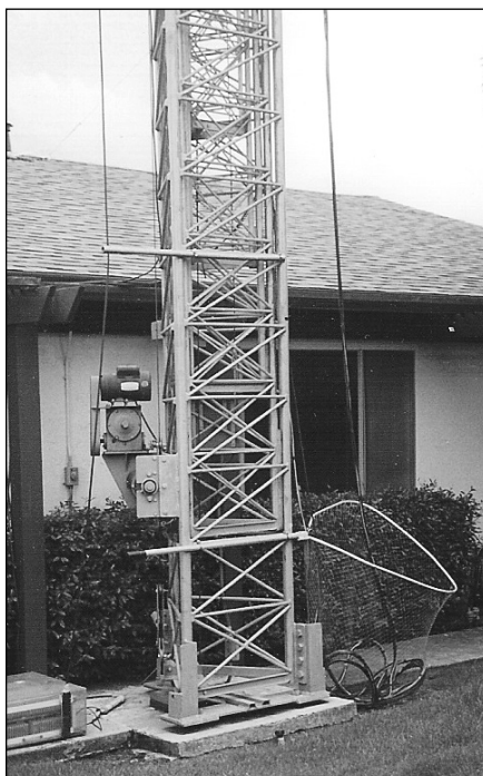
Figure 22.11 — The bottom of a crank-up tower is shown at left. The motor drive mechanism is on the left and a fishing net on the right catches and coils the feed lines and control cables as the tower is lowered. On the right, a fully loaded crank-up extended to its maximum height of 90 feet. [Steve Morris, K7LXC, photos]
