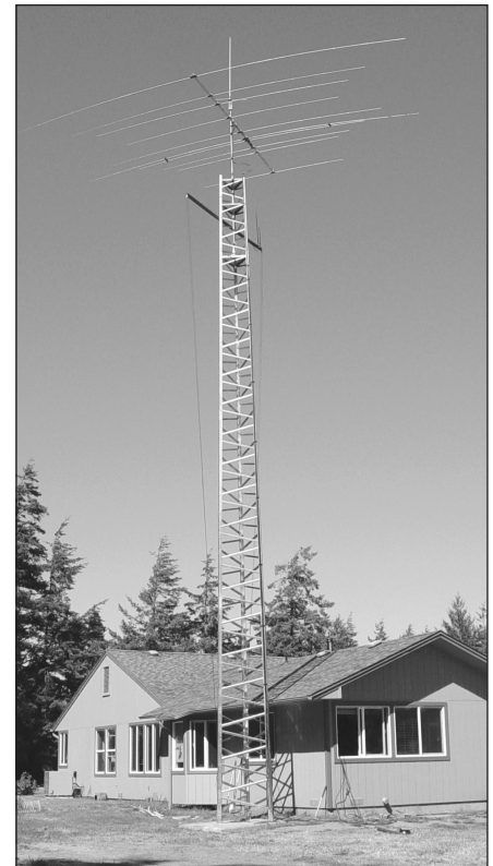
Figure 22.10 — A guyed tower with a good-sized load of antennas shown at the left. At the right, a Trylon Titan self-supporting tower. [Steve Morris, K7LXC, photos]
