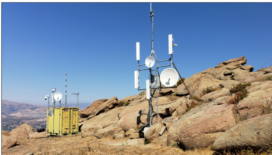
Figure 15.18 — A backbone site (right tower) in Southern California. User access points for 2 and 5 GHz are shown, along with a 5 GHz county backbone link. A 3 GHz local backbone node and a Part 15 wireless access point are also shown. (Photo courtesy Orv Beach, W6BI)
