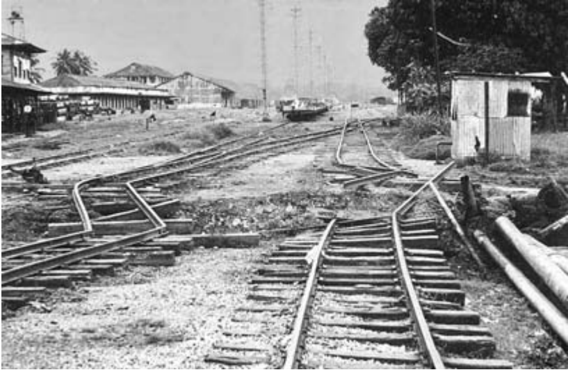
Figure 2.31 Bent rails near Gualán, Guatemala, after earthquake on 4 February 1976 from movement along the Motagua Fault, which marks the contact between the North American and the Caribbean plates (see fig. 2.30). Earthquakes result as the Caribbean plate slides eastward relative to the North American plate. From Espinosa 1976.
